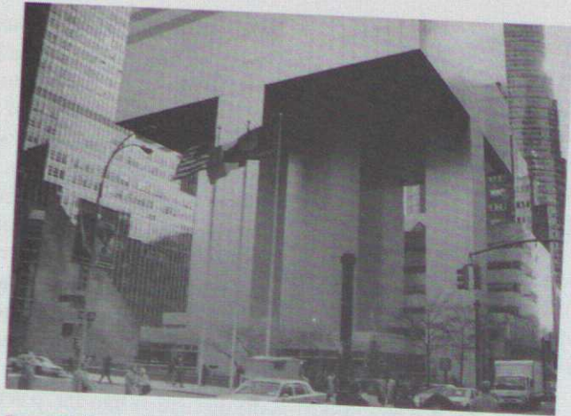
FIGURE 12.3 One view of the 59-story Citicorp Center, designed by architect Hugh Stubbins, Jr., with William J. LeMessurier serving as structural consultant. One of this building's notable features is that it rests on four massive columns that are placed at the midpoints of the building's sides, rather than at the corners. This enabled the architects to include under the Citicorp's sheltering canopy a new building for St. Peter's Church. (Photo by Clive L. Dym.)
